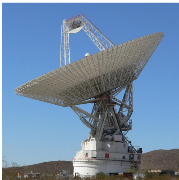
Figure 19.3 Radar Telescope. This dish-shaped antenna, part of the NASA Deep Space Network in California's Mojave Desert, is 70 meters wide. Nicknamed the "Mars antenna," this radar telescope can send and receive radar waves, and thus measure the distances to planets, satellites, and asteroids. (credit: NASA/JPL-Caltech)
